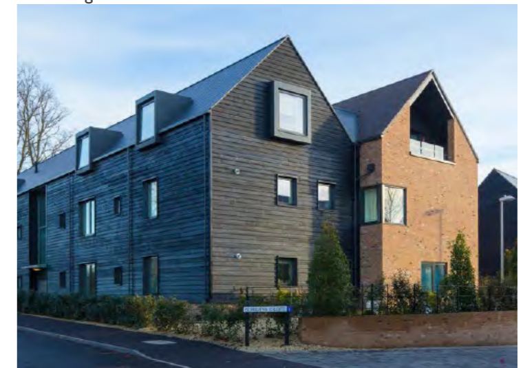
Apartment block form integrated with housing, The Avenue, Saffron Walden, by Pollard Thomas Edwards Architects.
