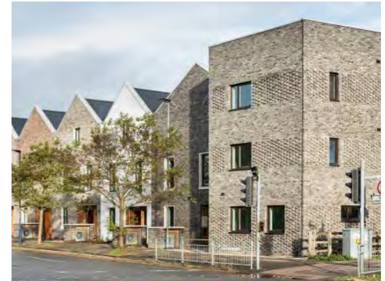
Apartment typology to address a key corner, Marmalade Lane, Cambridge. Mole Architects.
