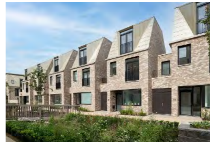
Broken terrace with integrated parking, Knights Park, Eddington, by Alison Brooks Architects.
