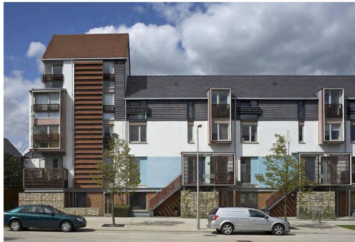
Extra floor to provide height landmark at Abode, Newhall, Harlow by Proctor and Matthews Architects.
