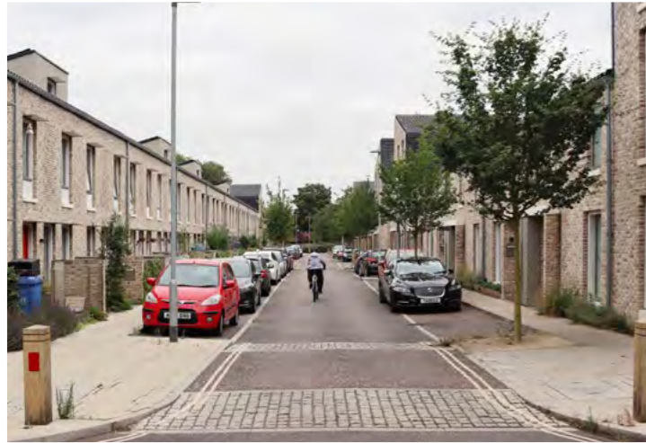
Local Street example at Goldsmith Street, Norwich. Mikhail Riches Architects.
