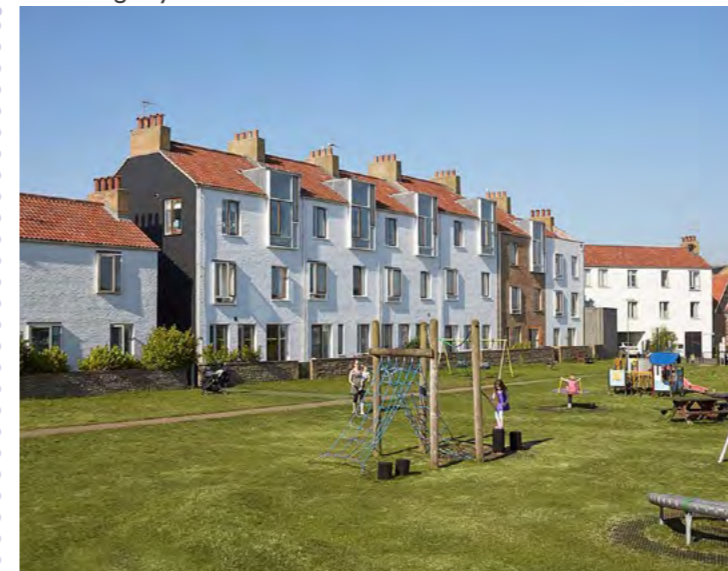
Example of landmark frontage to key open space, Southwold, by Ash Sakula Architects.
