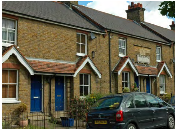
Articulated windows on Oddfellows Terrace, Old Harlow.
